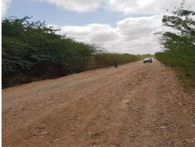
Figure 10 Left: View of Dolow Road, Right: Blocked culvert inlet
