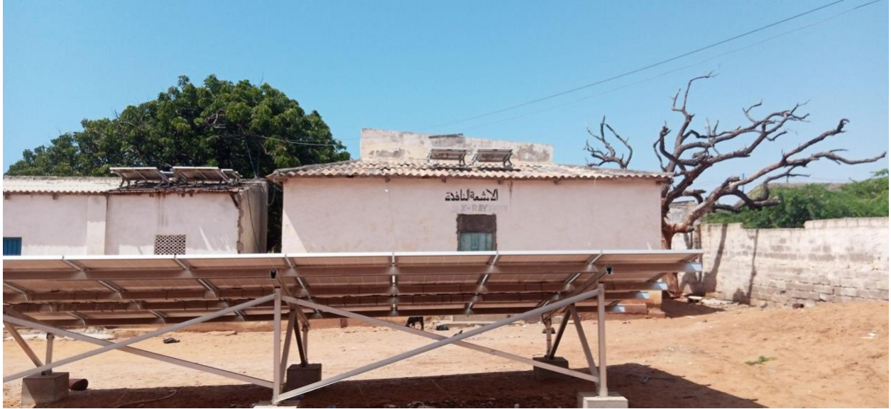
Figure 4-2: Current TB unit buildings with solar panels to the foreground
