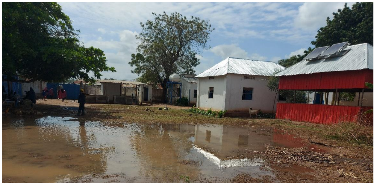
Figure 3-6: current Kulmis MCH, waiting area in red iron sheets, under 5 clinic to the right and the laundry area, pit latrine and entrance in the background
