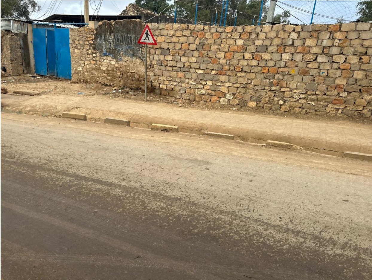
Image 5-5: View of drainage channel next to the project site
