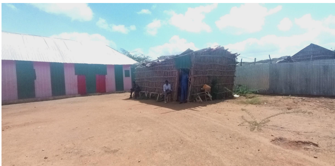
Figure 39: The current Horseed HF waiting room
