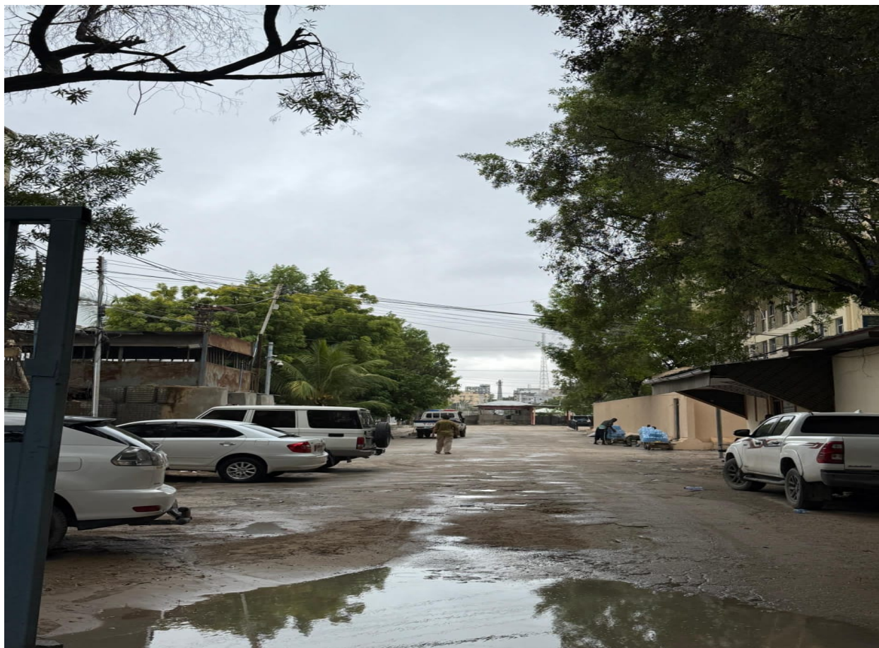
Figure 6: View of stagnant water on the ministry HQ compound
