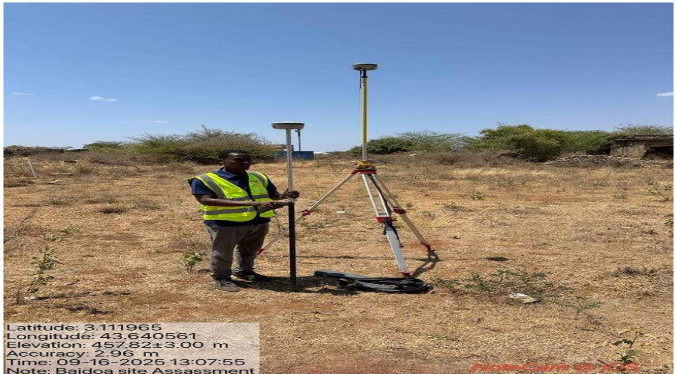
Figure 1 Baidoa CSC office site photo during engineering assessment
