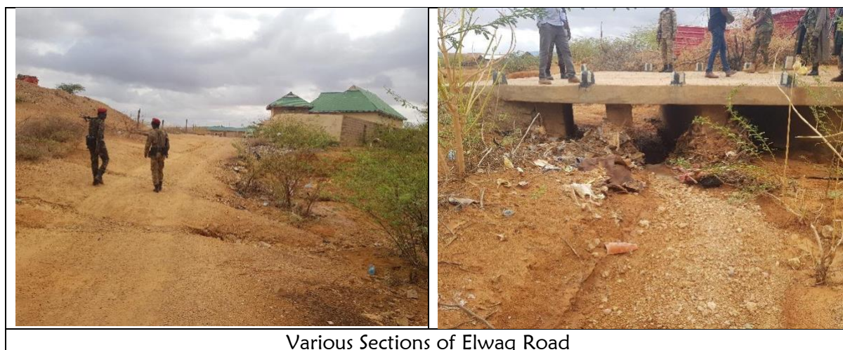
Figure 2: Various Sections of Elwaq Road
